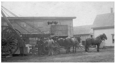
Galamanders were used to transport large pieces of granite using teams of oxen or horses. These wagons were equipped with a boom and would carry the granite slung underneath the large rear wheels. According to Sidney Winslow's book *Fish Scales and Stone Chips*, the iron work was done by Charles Littlefield at the Bodwell Granite Company's job shop on Main Street. At the time of Winslow's
